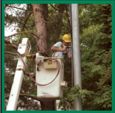
Apprentice Lineman Jarred Martens secures the pole guard on a service during a system improvement job, one of many projects designed to make the system more reliable for you.
